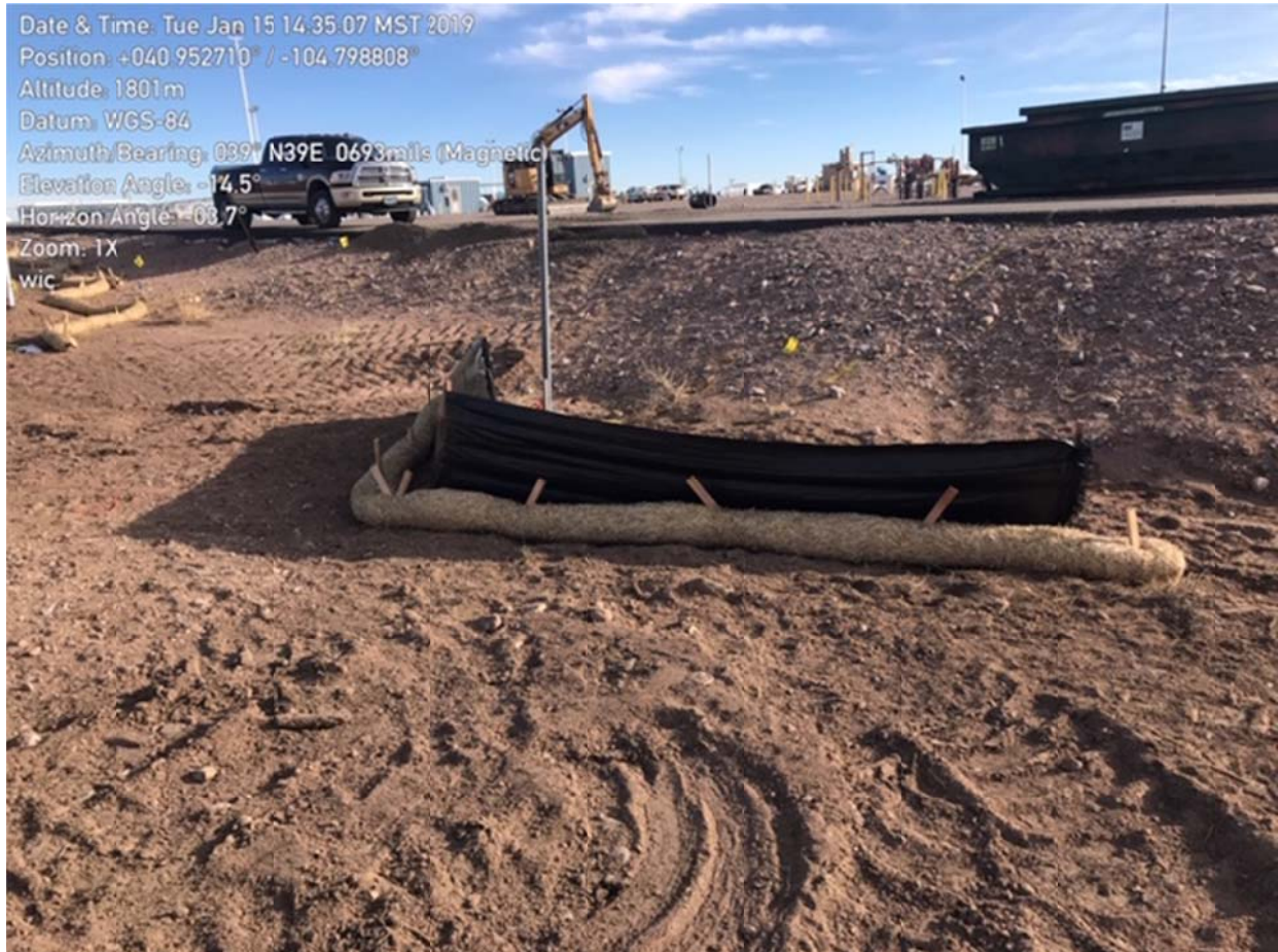
Installation of final erosion control device south of the scrubber vessel work area
