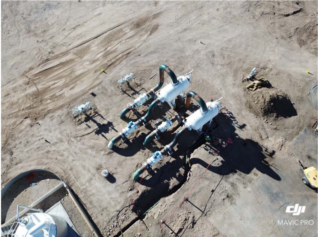
Backfill mostly complete at the scrubber vessels
