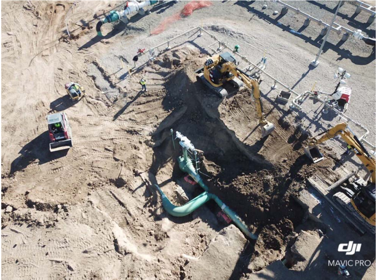
Backfilling the tie-in at the Flying Hawk Meter Station
