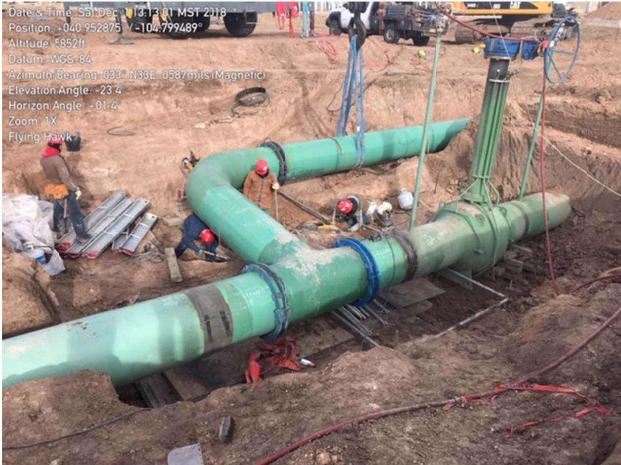
Flying Hawk Meter Station tie-in
