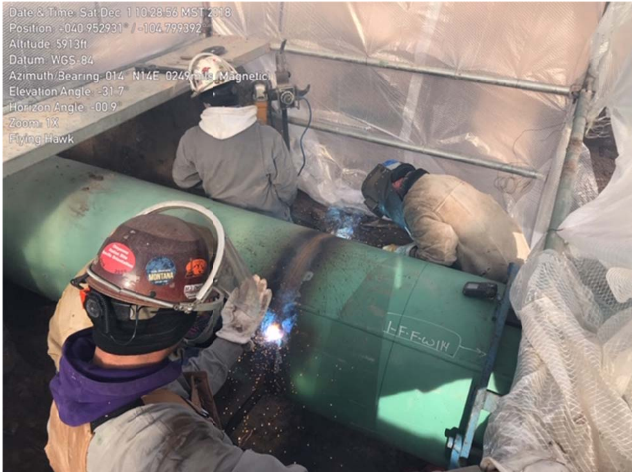
Tie-in weld at the Flying Hawk Meter Station
