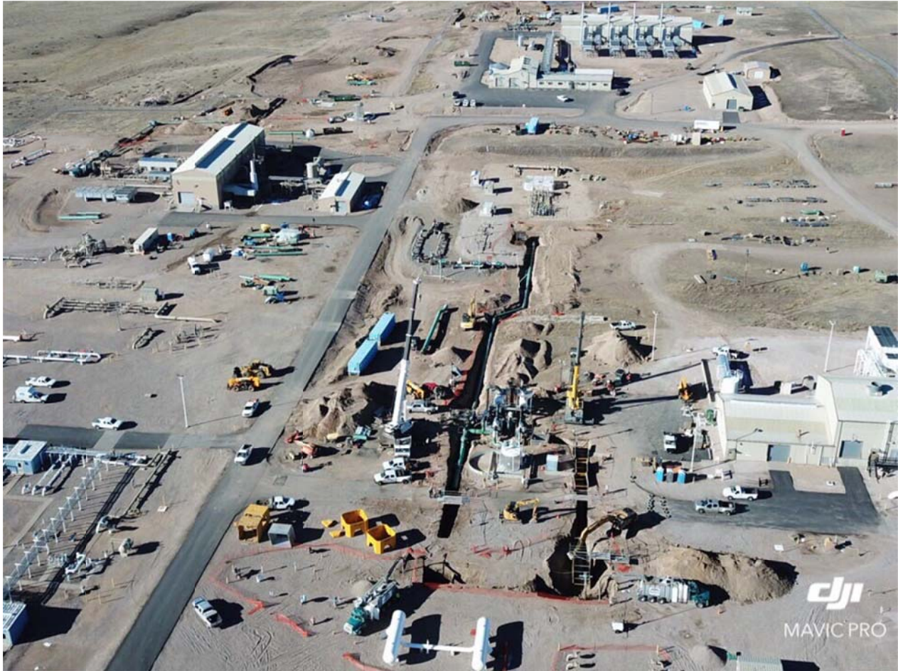
Overview of connecting pipeline between Flying Hawk Meter Station and WIC compressors
