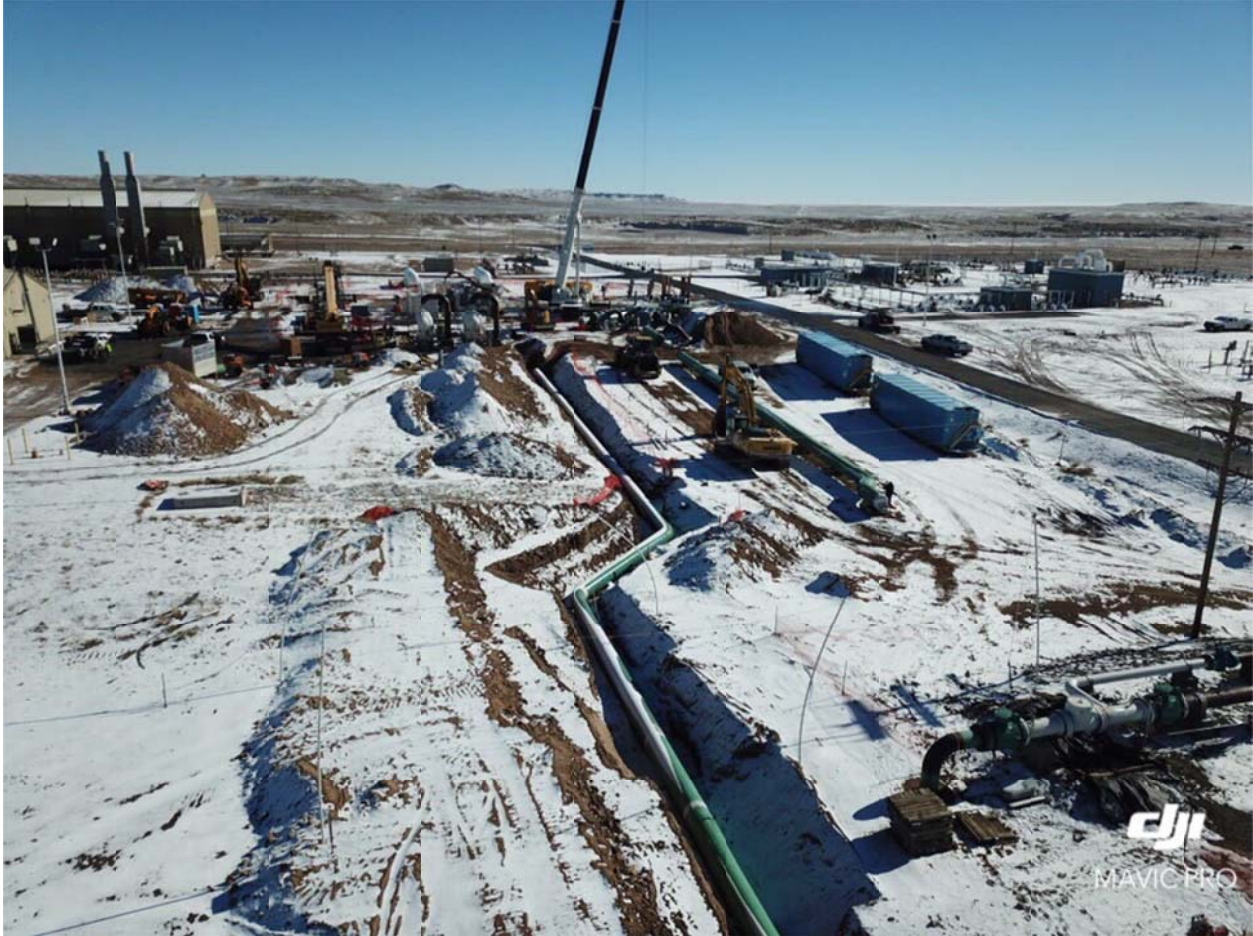
Plant-yard piping installed
