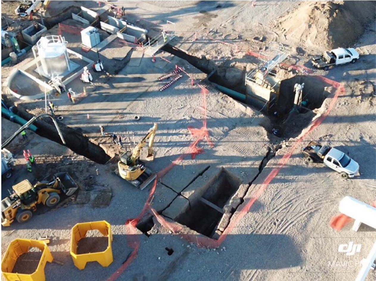
Excavation for the WIC compressor suction line tie-ins
