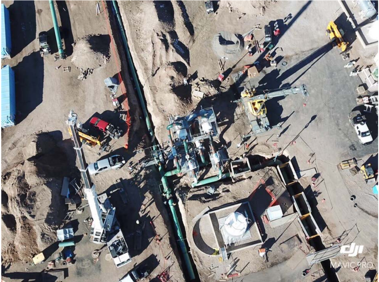
Installation of trench boxes at the WIC compressor suction tie-in
