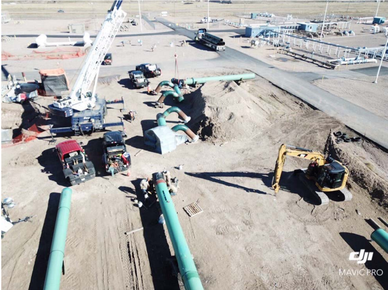
Fabrication work at the scrubber vessel site
