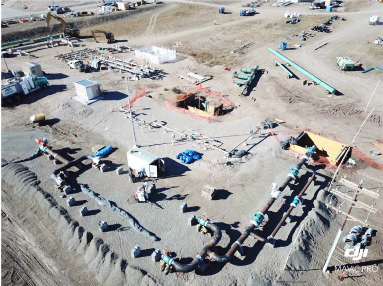
Sparrow Meter Station
