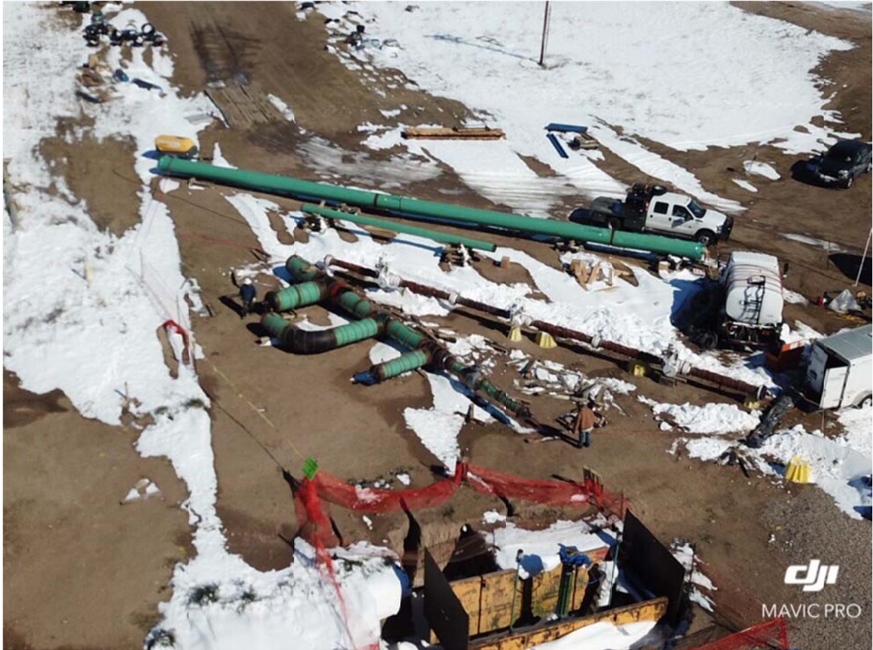
Hydrostatic test area
