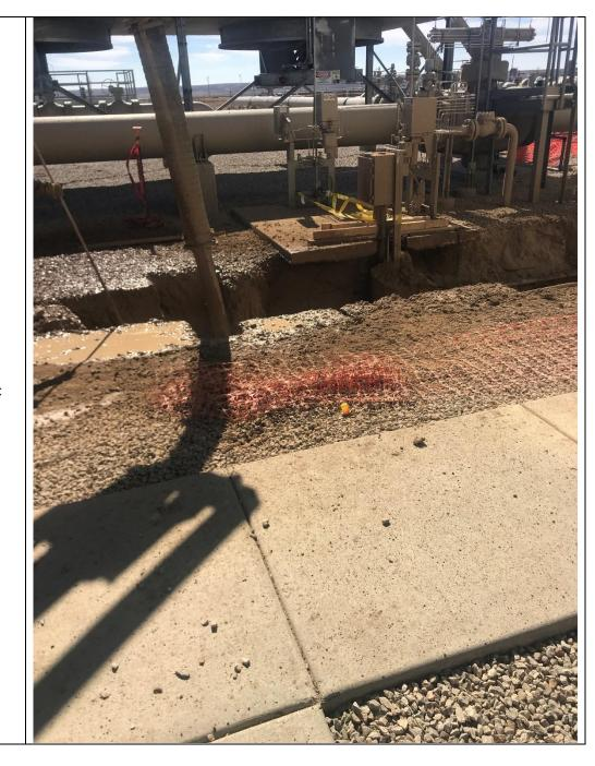
Location: Wamsutter Compressor Station Direction of Photo: West Description: Hydrovac operations for the temporary silencer. Date: 10/05/2024 Location: Wamsutter Compressor Station Direction of Photo: West Description: Auxiliary building foundation excavation completed. Date: 10/07/2024
