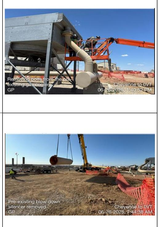
Location: Wamsutter Compressor Station Direction of Photo: Northwest Description: Removal of existing blowdown silencer. Date: 6/26/2025
