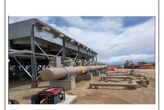
Location: Wamsutter Compressor Station Direction of Photo: West Description: Removing water from hydrostatic test. Date: 5/16/2025
