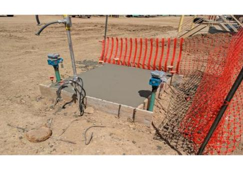
Location: Wamsutter Compressor Station Direction of Photo: East Description: Poured concrete pad for emergency shut down panel. Date: 5/9/2025
