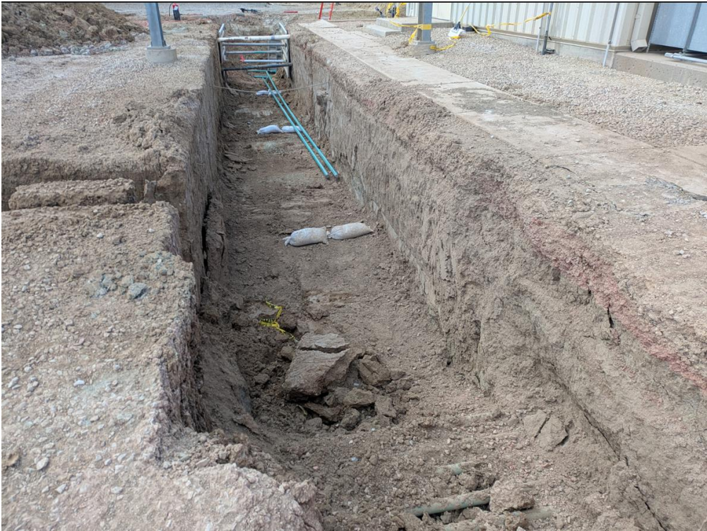
Location: Wamsutter Compressor Station Direction of Photo: N/A Description: Installing 2-inch emergency shut down lines. Date: 3/13/2025
