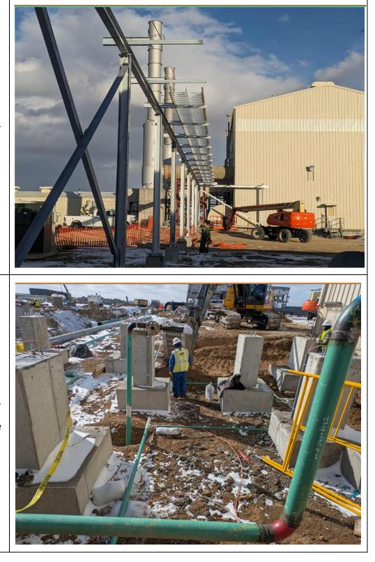
Location: Wamsutter Compressor Station Direction of Photo: N/A Description: Backfilling the supports behind the engine room. Date: 2/14/2025
