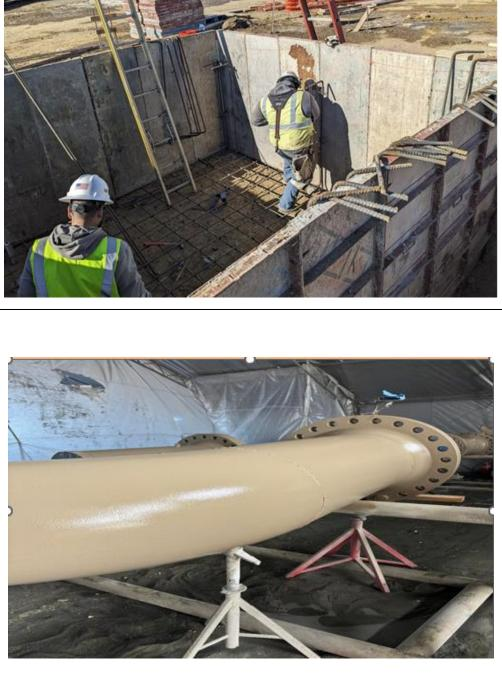
Location: Wamsutter Compressor Station Direction of Photo: N/A Description: Topcoat completed on fabrication. Date: 1/29/2025 Location: Wamsutter Compressor Station Direction of Photo: N/A Description: Excavation for the 24-inch discharge line. Date: 1/30/2025
