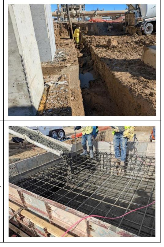
Location: Wamsutter Compressor Station Direction of Photo: N/A Description: Pouring concrete for the silencer foundation Date: 1/31/2025
