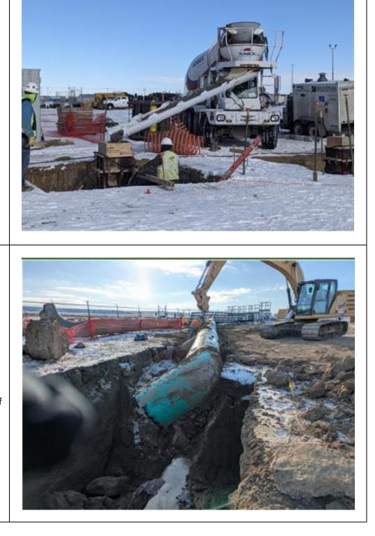
Location: Wamsutter Compressor Station Direction of Photo: South Description: Removal of the last section of 36inch demo pipe. Date: 1/16/2025
