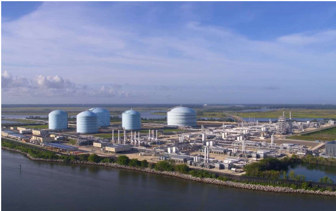
Elba Island LNG Import/Export Facility All liquefaction equipment is electric drive
