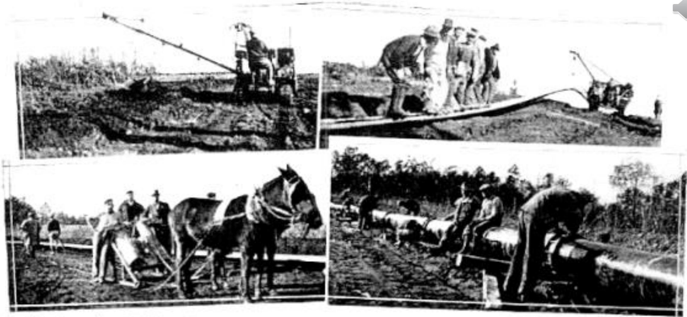
Top, left: A machine of this description can backfill in the course of a day from 6,000 to 7,000 linear feet of trench—doing work that would require a large force of men. Right: Method employed in making a “cold head” in an 8-inch welded line.
