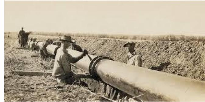
Combination of coupled and acetylene welded pipe
