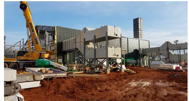
Broad Run Expansion – Sta. 563 Construction
