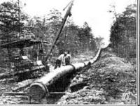
(1) One of the few teams used on the project with view of line approaching creek bed. (2) Pipe line crossing on concrete paving, showing crossing undisturbed. (3) Ditch ready for pipe. (4) Section of pipe, with Dresser couplings ready to be lowered into excavation.
