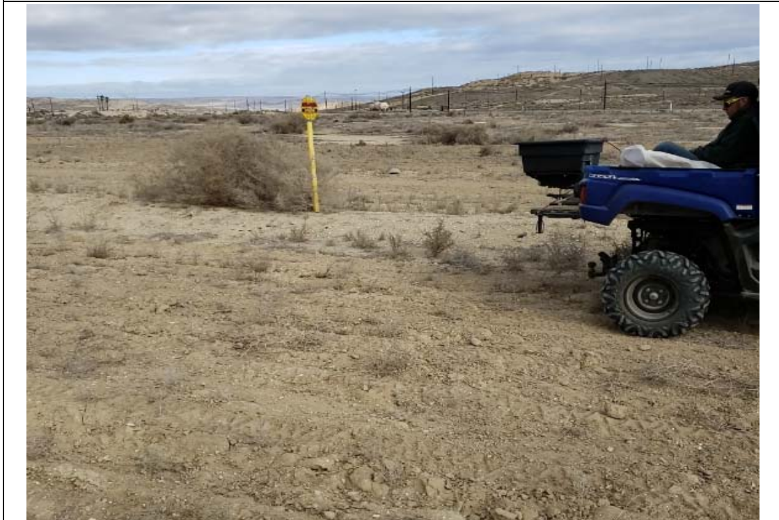
Photo No. 4: Line 1901 Replacement Project, Kern County, California
