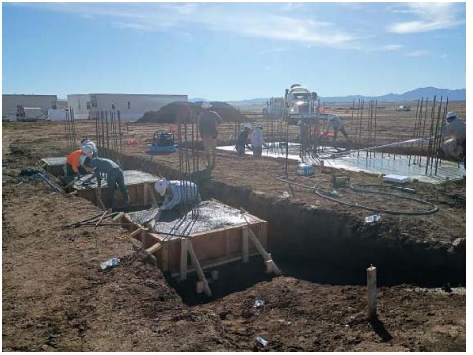
A photograph showing several construction workers in hard hats and safety vests pouring concrete into large, rectangular foundation forms. The forms are supported by vertical rebar. In the background, a concrete mixer truck is parked, and the surrounding area is a dry, open landscape with some distant buildings.                                                                                              |
