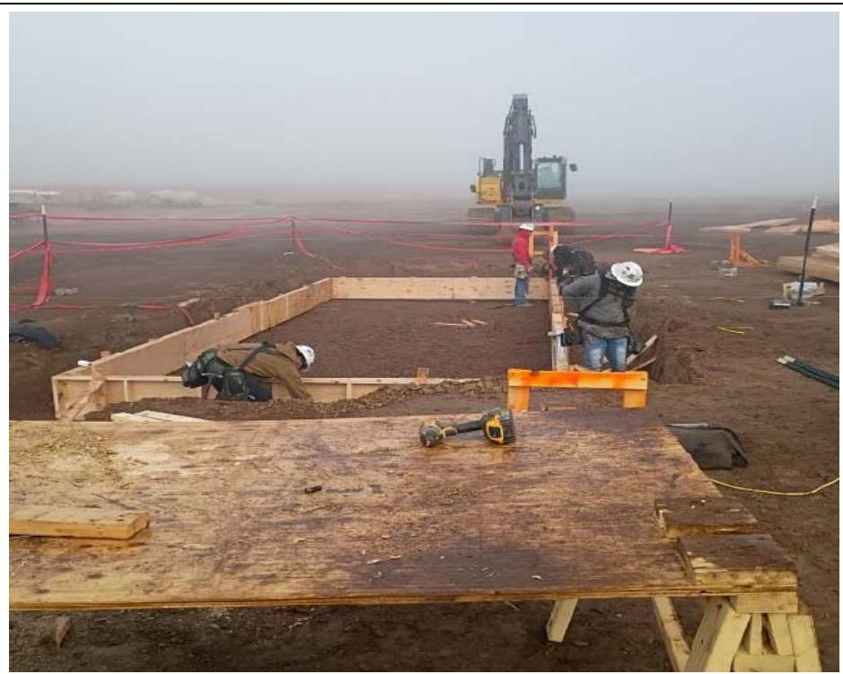
A photograph showing construction workers setting forms for cooling tower supports. The workers are wearing hard hats and safety vests. One worker is kneeling on the ground, another is standing. They are working on a wooden form structure. In the background, there is a yellow excavator and a large construction site under a clear sky. |
