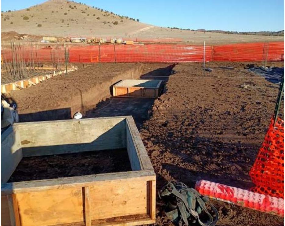
A photograph showing the construction of wooden forms for gas cooler supports. The forms are made of yellow wooden boards and are being used to create a large, rectangular concrete structure. In the foreground, a red safety tape is visible. The background shows a dirt construction site with a red fence and a hill in the distance under a clear blue sky. |
