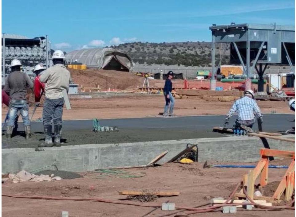
A photograph showing several construction workers in hard hats and safety vests pouring concrete onto a foundation. The workers are using long-handled tools to spread the concrete. In the background, there are large industrial structures, including a large grey building and a green tent-like structure. The sky is clear and blue. |
