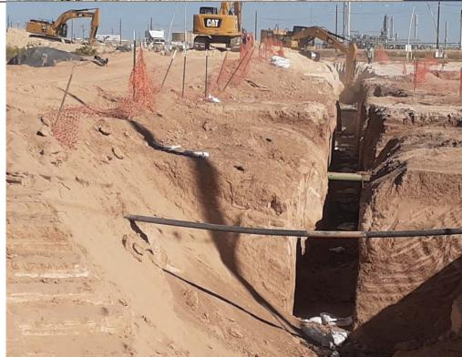
Number 578+00 **Direction of Photo:**Northwest **Description:** Silt fence installed on edge of ROW, topsoil pile stabilized with hay, and excavated trench. **Date:** 10/16/2020
