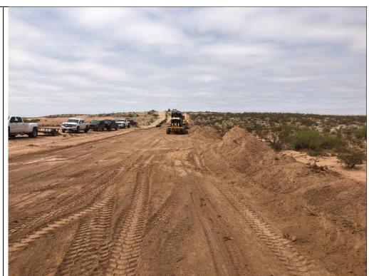
Location: Station No. 860+00, Temporary Access Road 2 Direction of Photo: North Description: Track hoe assisting with installation of erosion control devices.
