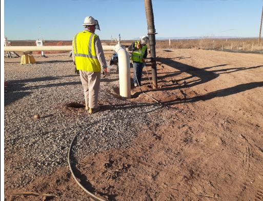
Location: Station Number 465+00 Direction of Photo: East Description: View of an operator padding the pipeline trench. Date: 01/07/2021
