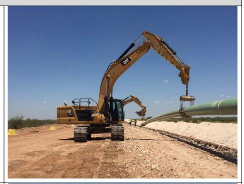
Location: Line No. 31111 ROW at Station No. 701+00 Direction of Photo: North Description: Open ditch prepped for pipe lowering in.
