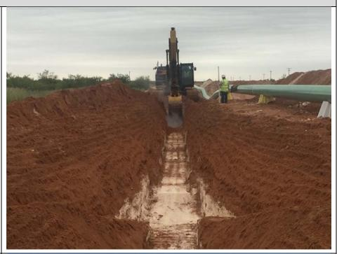
Location: Line No. 31111 ROW at Station No. 256+00 Direction of Photo: Southwest Description: Digging out the bore pit on the south side of County Road 107.
