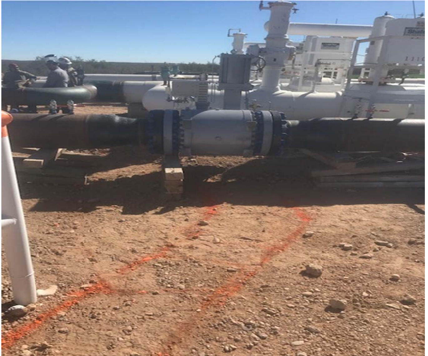
Photo No. 1 – New back pressure valve on Line No. 1110 at Pecos River Compressor Station
