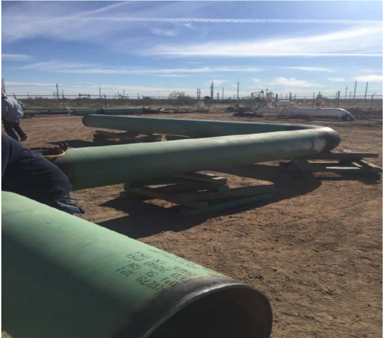
Photo No.3 – Fabricated pipe to be installed on Line No. 1115 following hydrostatic testing
