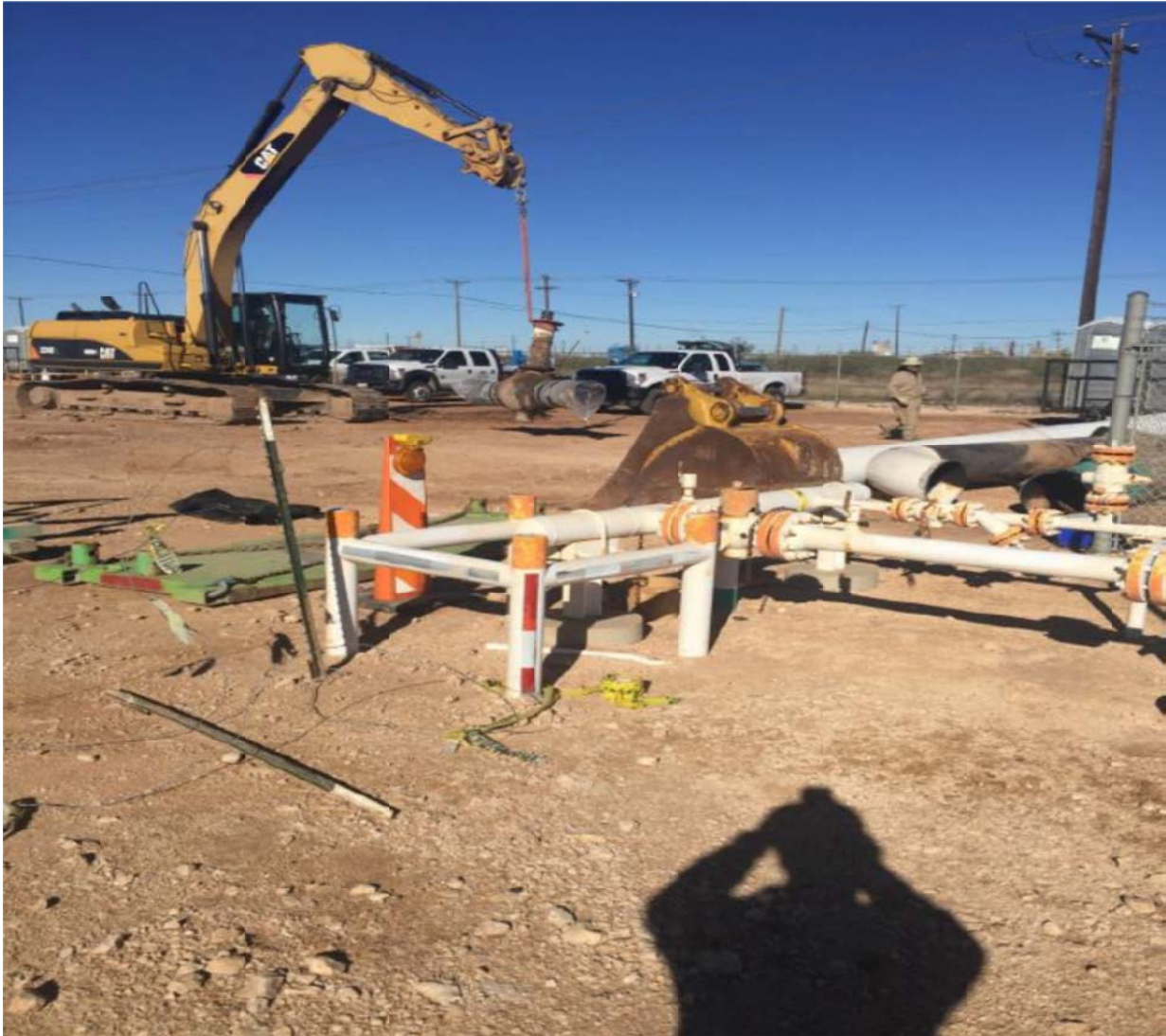
Photo No. 4 – Removal of scrap pipe and clean-up activities on section of Line No. 1115
