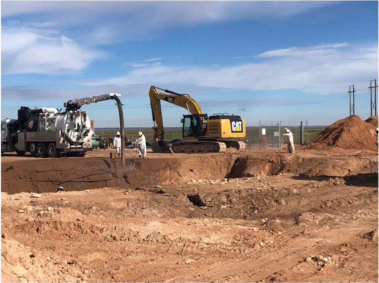
Photo No. 4 – Hydrovac activities at Eunice Compressor Station.
