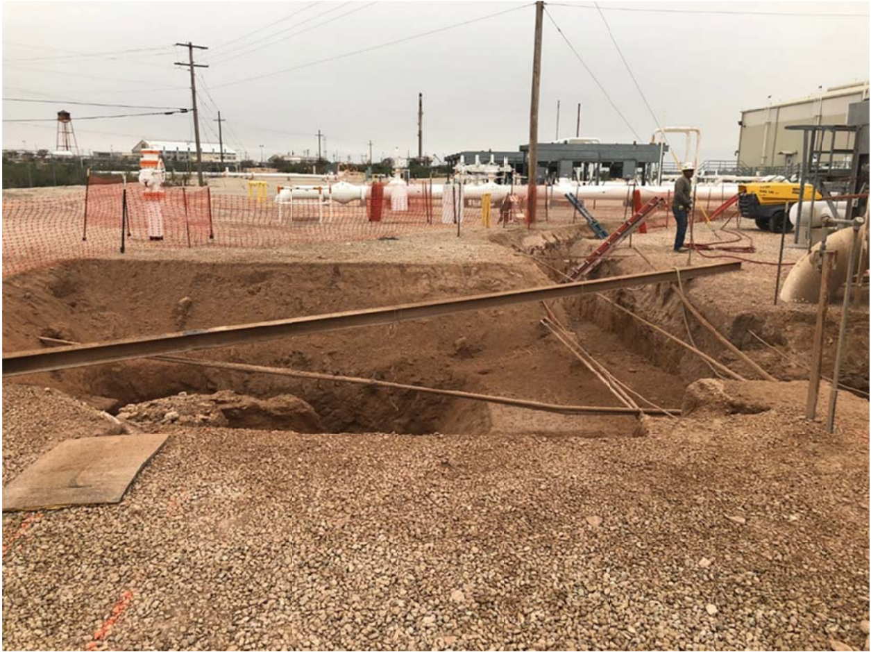
Photo No.3 – Hydrovac activities at Eunice Compressor Station.
