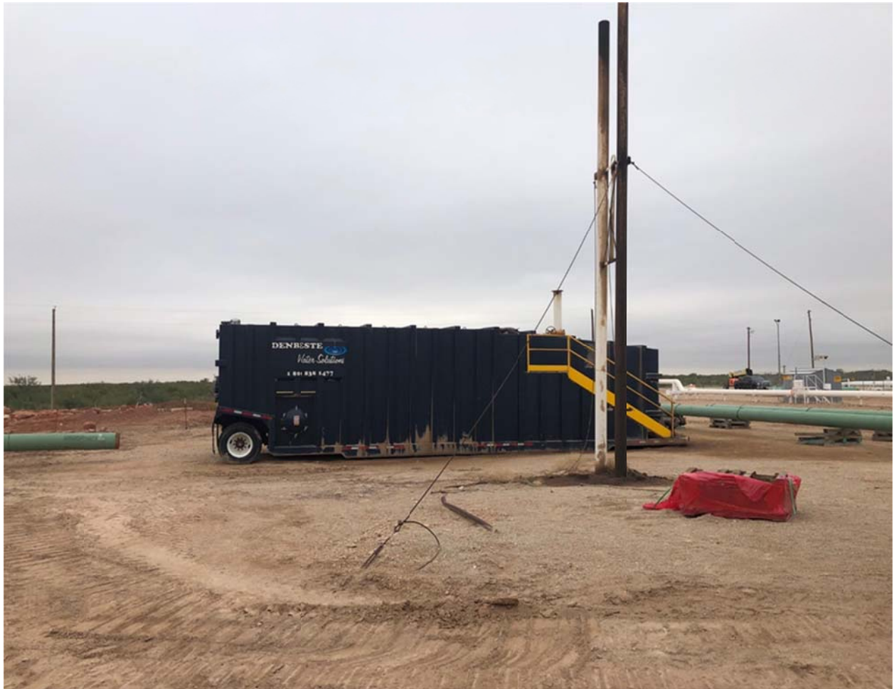
Photo No. 2 – Tank holding hydrostatic test water at Line No. 1115 work location.
