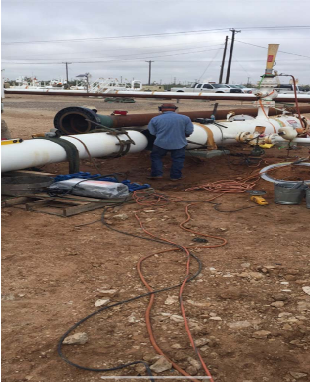
Photo No. 1 – Preparing Line No. 1115 for hydrostatic testing.
