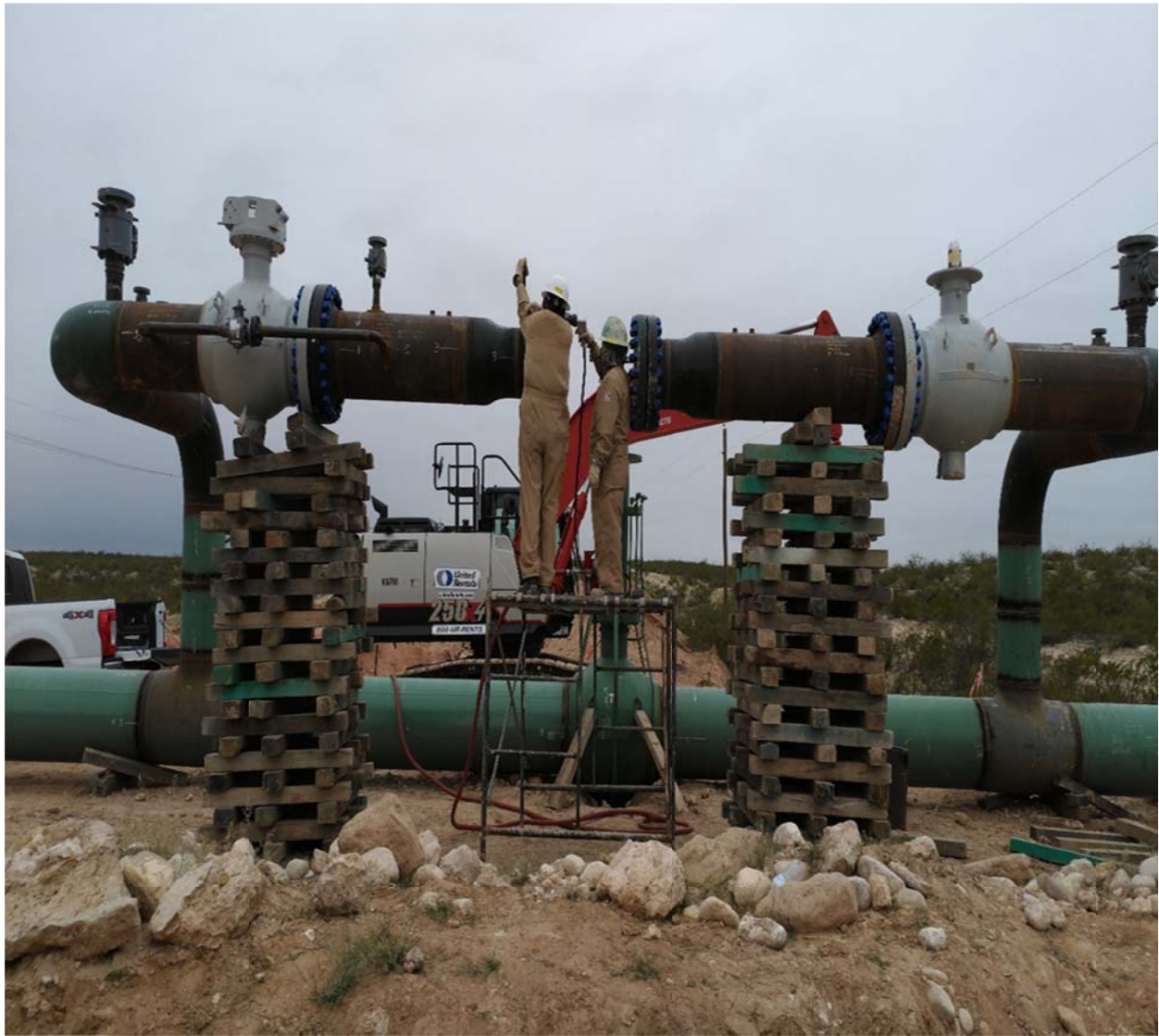
Photo No. 4 – Preparing for hydrostatic testing at the Ramsey North Meter Station.
