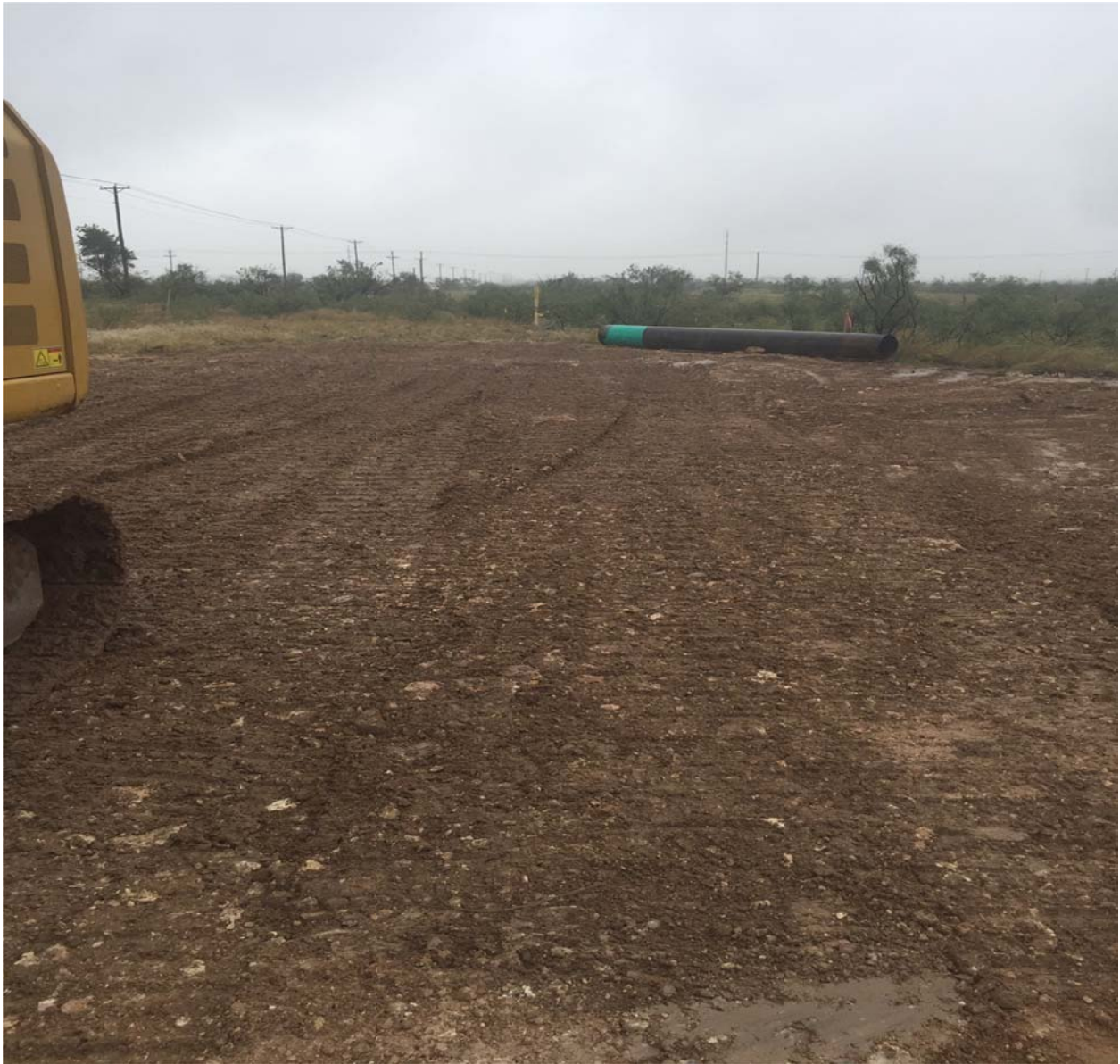
Photo No. 2 - Cleanup activities on Line No. 1115 work location.
