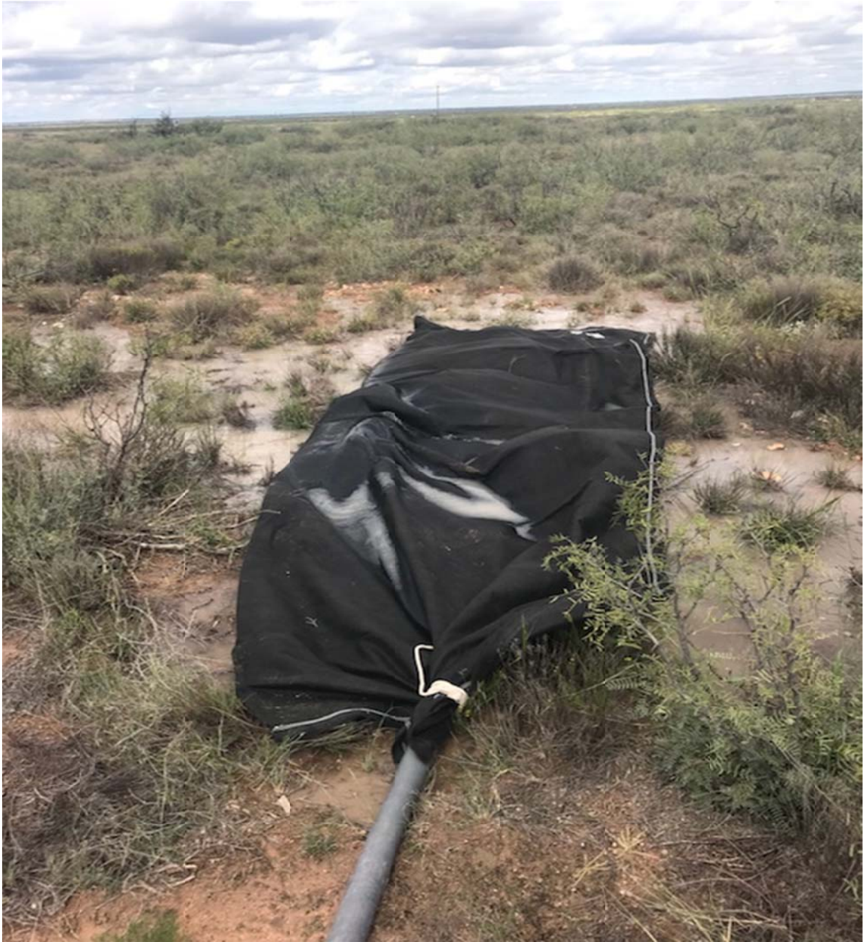
Photo No. 1 – Pumping out ditch water at Eunice Station with approved filter bag.
