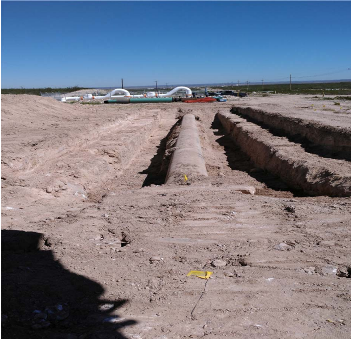
Photo No. 4 – Exposing pipe at the Ramsey North Meter Station.
