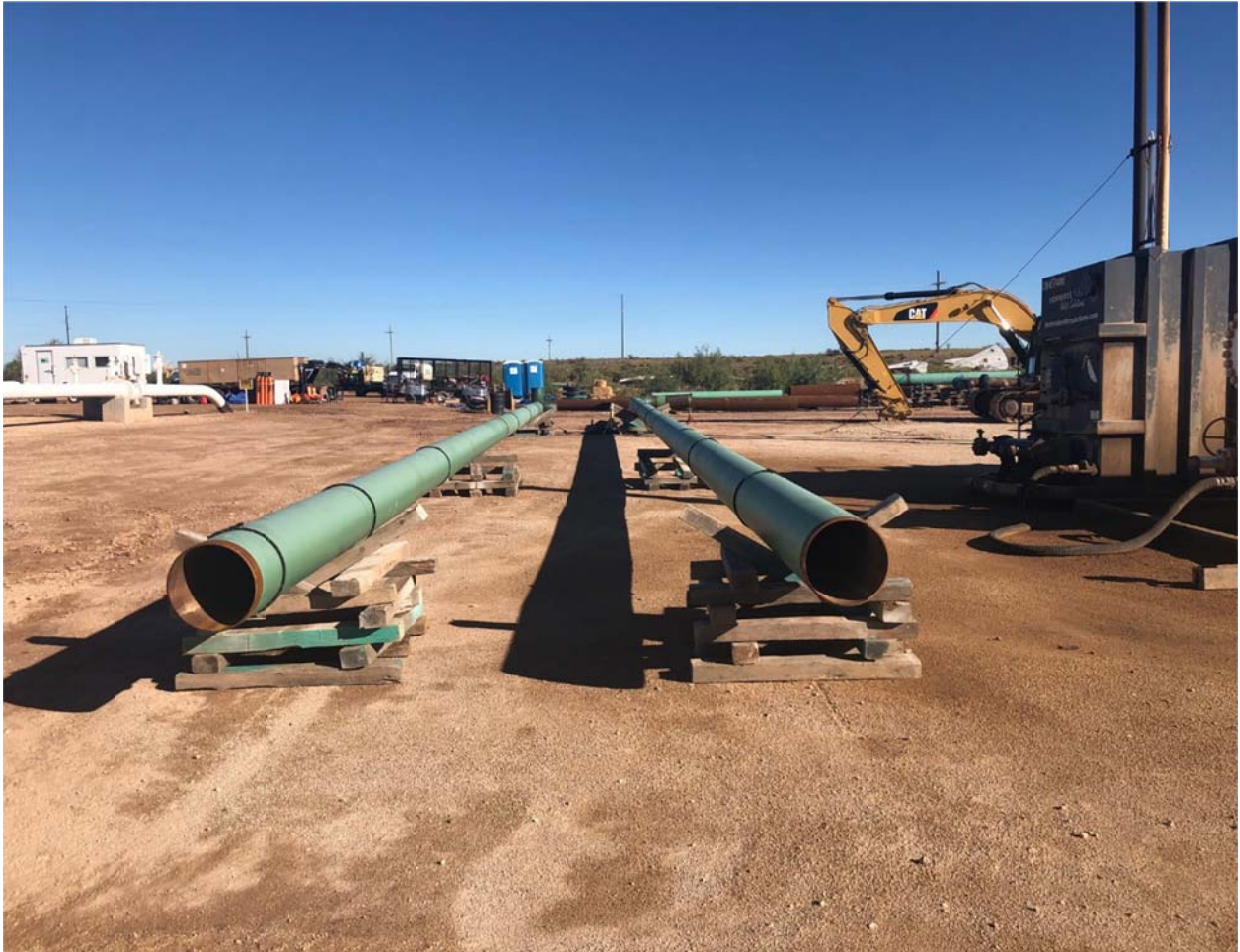
Photo No.3 - Contractor prepping for hydrostatic testing at Pecos River Compressor Station.
