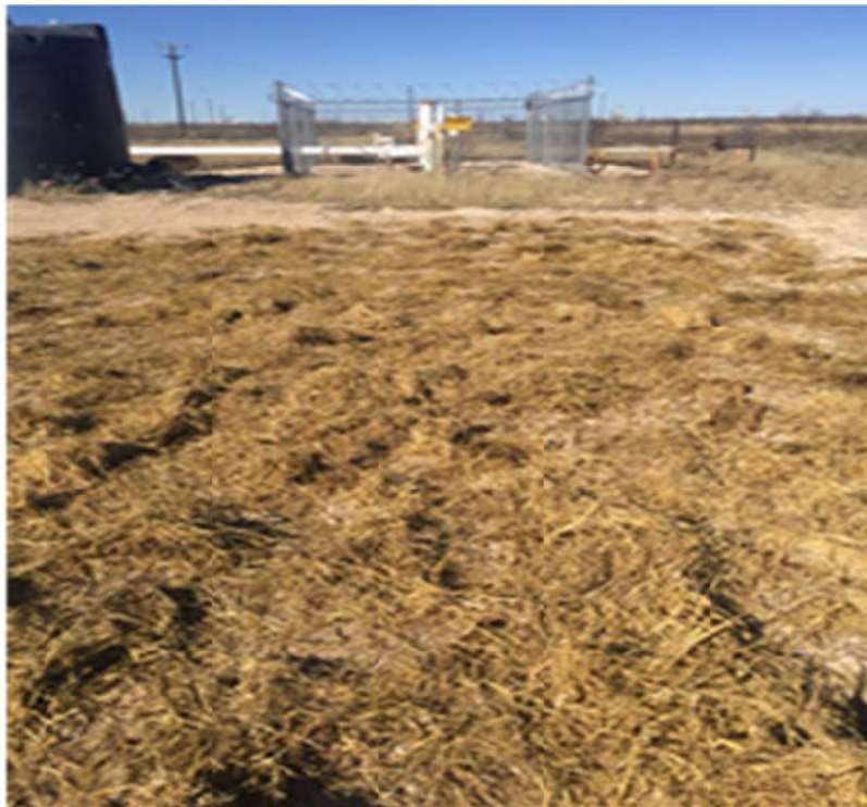
Photo No. 2 – Line No. 1115 work location reseeded and mulched.
