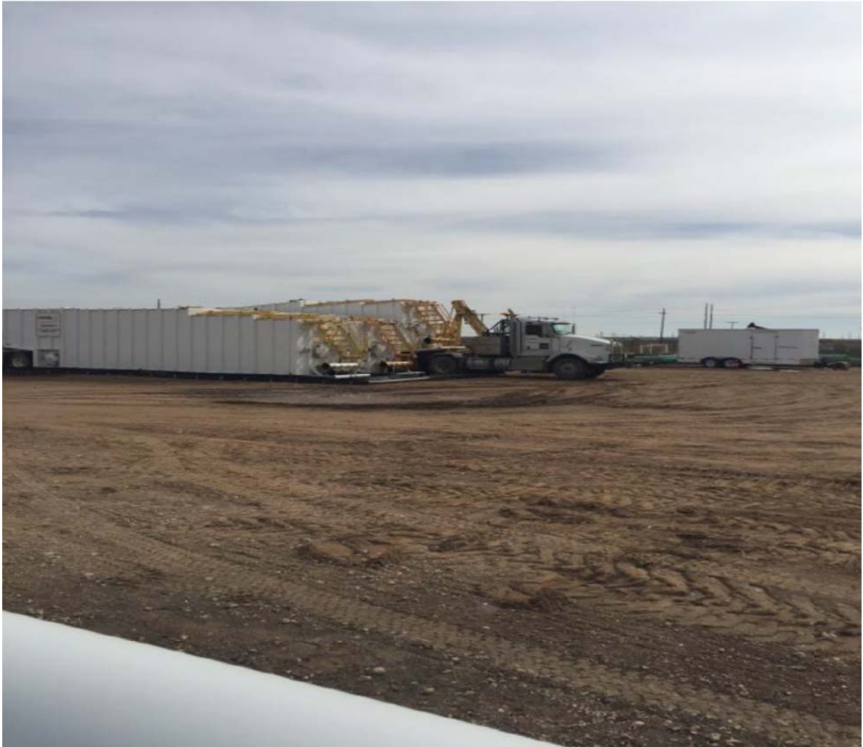
Photo No. 1 – Removing frac tanks from the Line 1115 hydrostatic pressure test location
