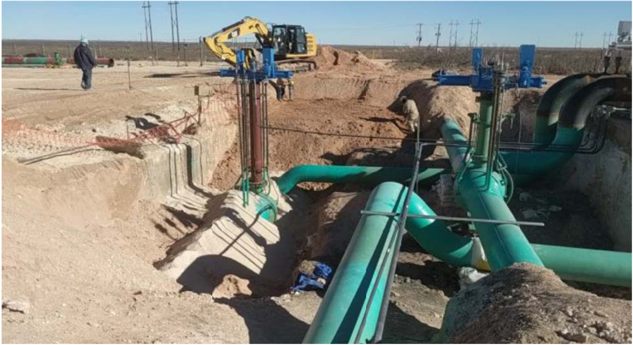
Photo No. 3 – Backfilling and compacting excavations at Eunice Compressor Station
