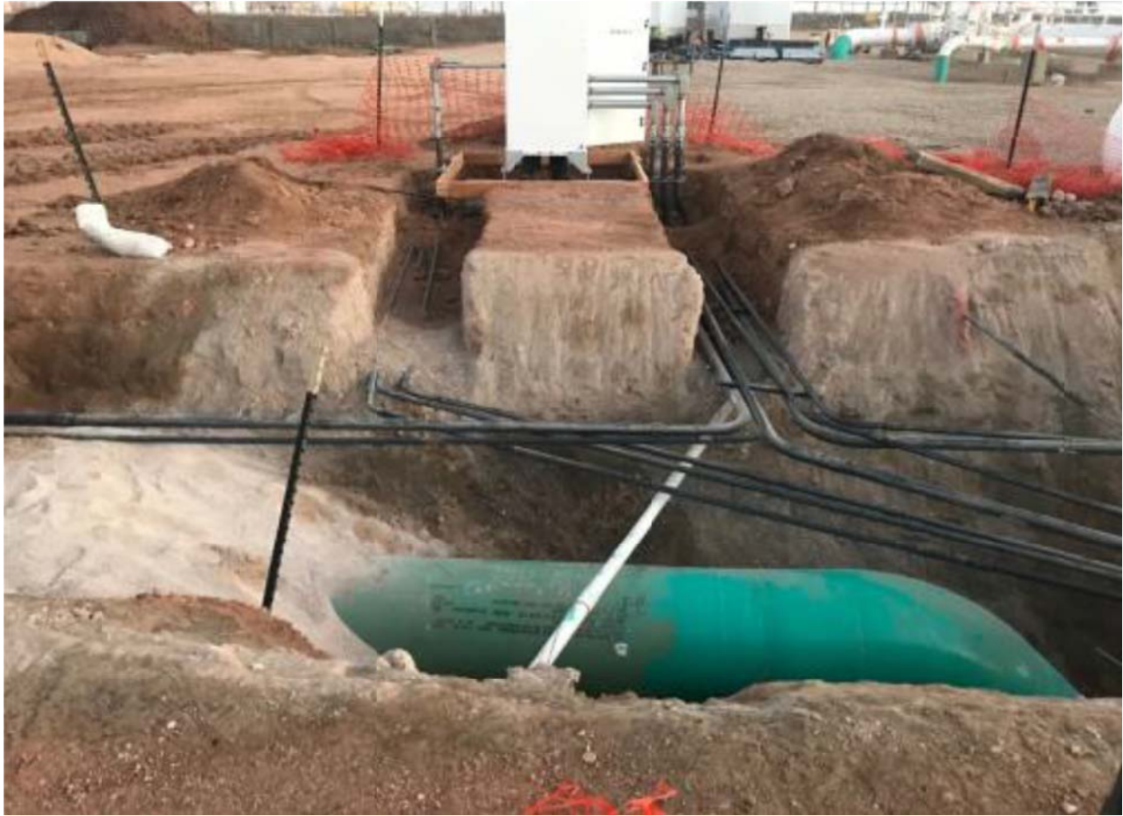
Photo No. 2 – Beginning backfill activities of excavations at Eunice Compressor Station
