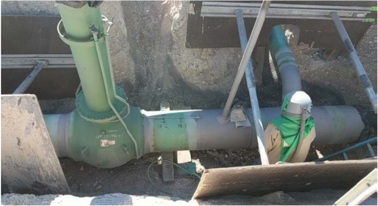
Photo No. 6 – Sandblasting pipeline at the Line No. 1119 isolation location
