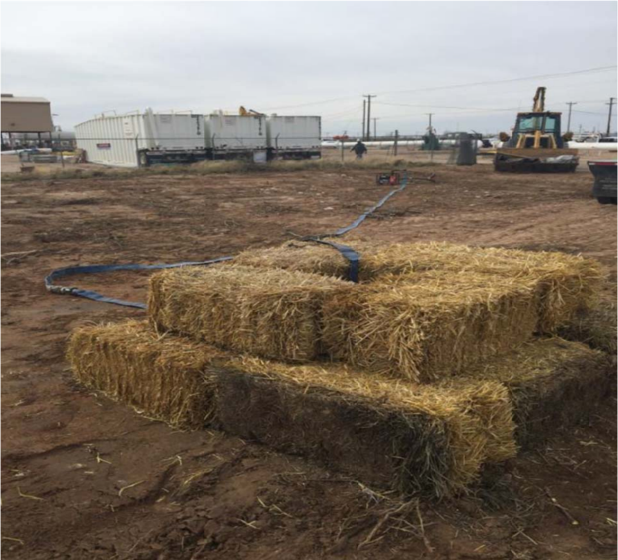
Photo No. 2 – Energy dissipation structure for discharged water at Line 1115 location
