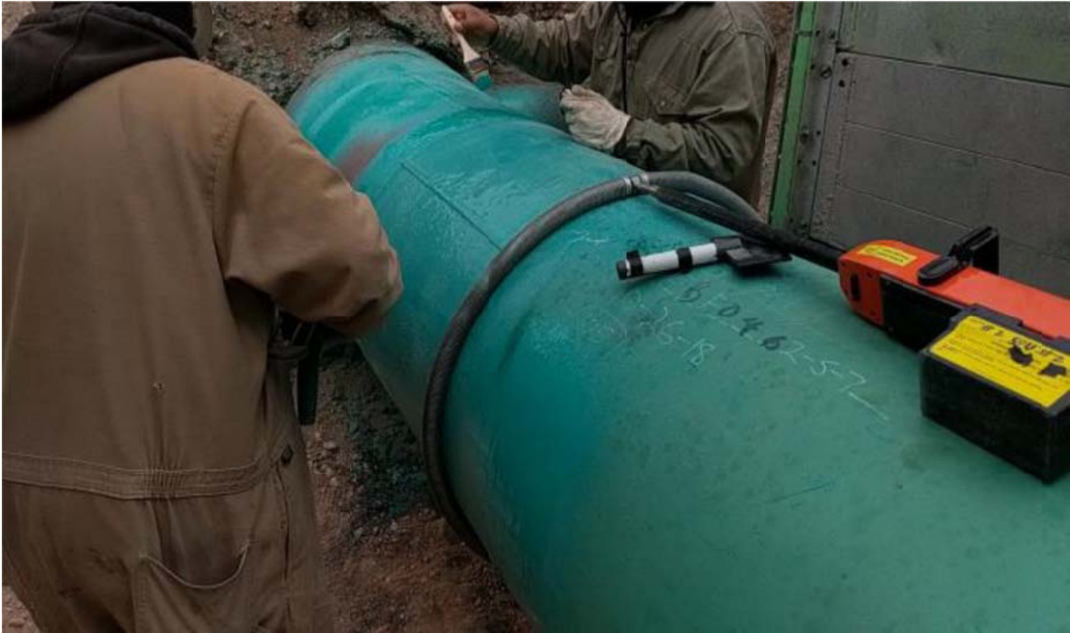
Photo No. 3 – Crews completing coating activities at Eunice Compressor Station
