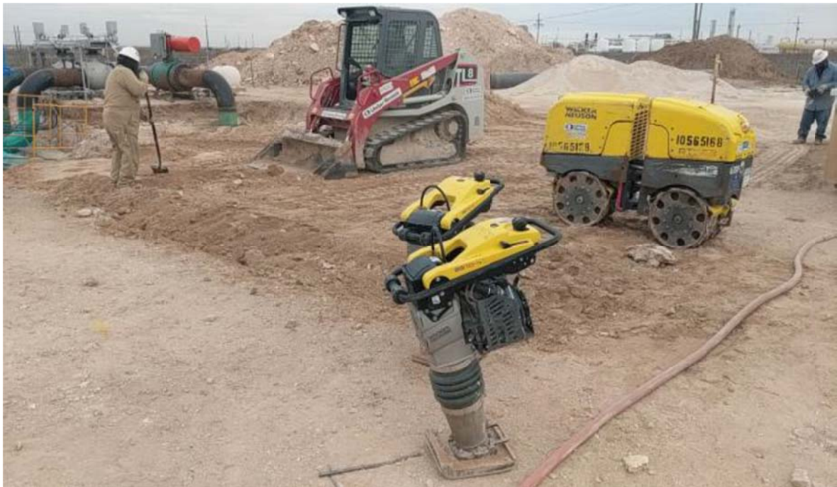
Photo No. 4 – Compacting the backfilled trench at Eunice Compressor Station
