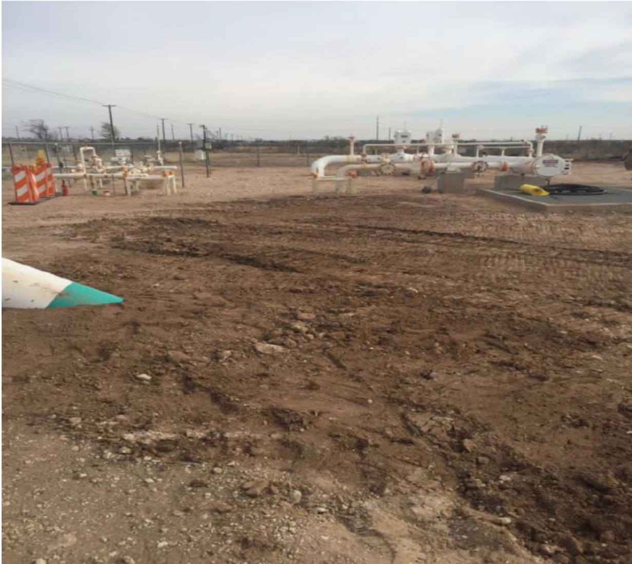
Photo No. 1 – Completed painting and backfill at Line 1115 hydrostatic pressure test location
