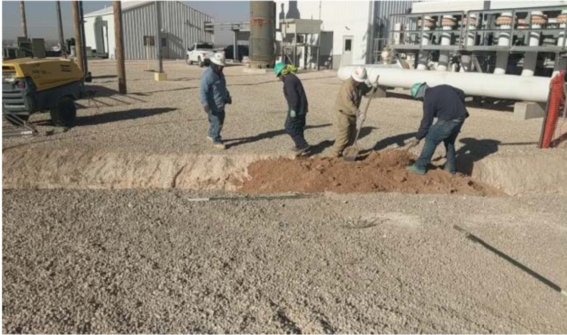
Photo No. 3 – Crews backfilling electrical conduit trench at Eunice Compressor Station
