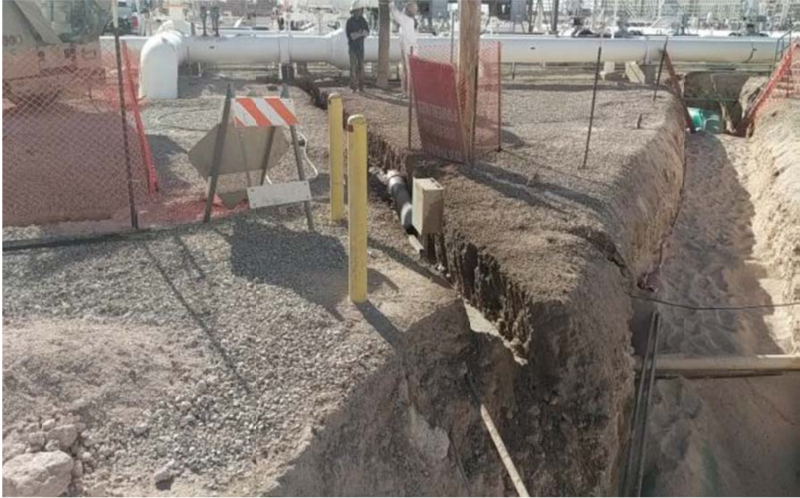
Photo No. 1 – Placement of electrical conduit at the Eunice Compressor Station
