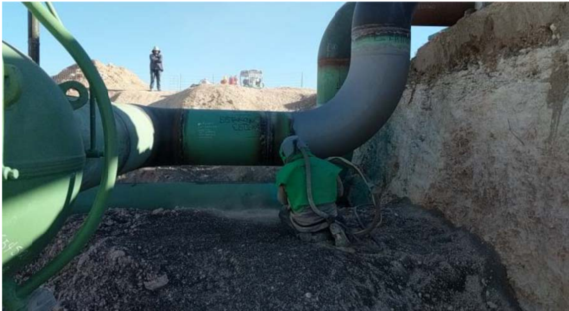
Photo No. 2 – Sand blasting below grade piping at the Eunice Compressor Station
