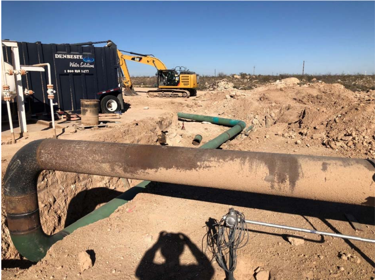
Photo No. 4 – Connecting new station crossover piping at Pecos River Compressor Station
