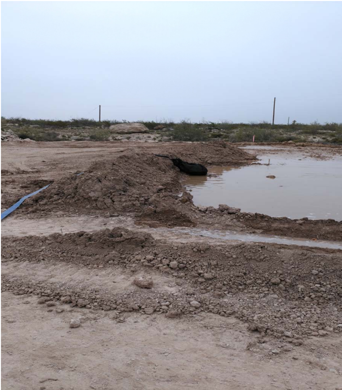
Photo No. 1 – Dewatering in an upland area within the Pecos River Compressor Station
