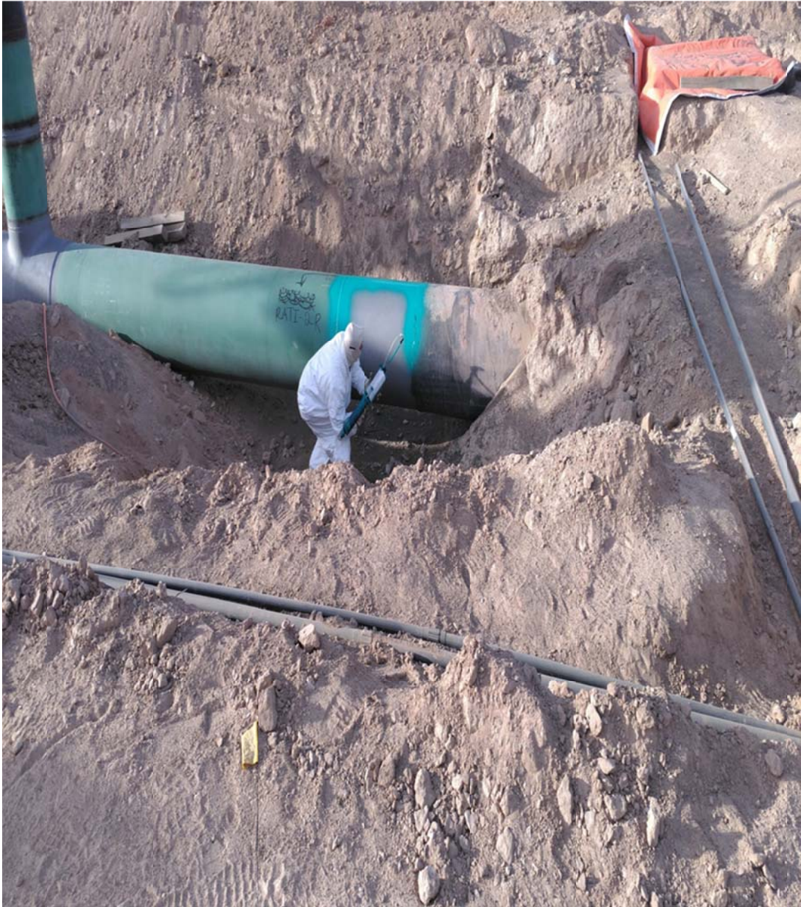
Photo No. 4 – Sandblasting and coating new valve installation at Ramsey North Meter Station
