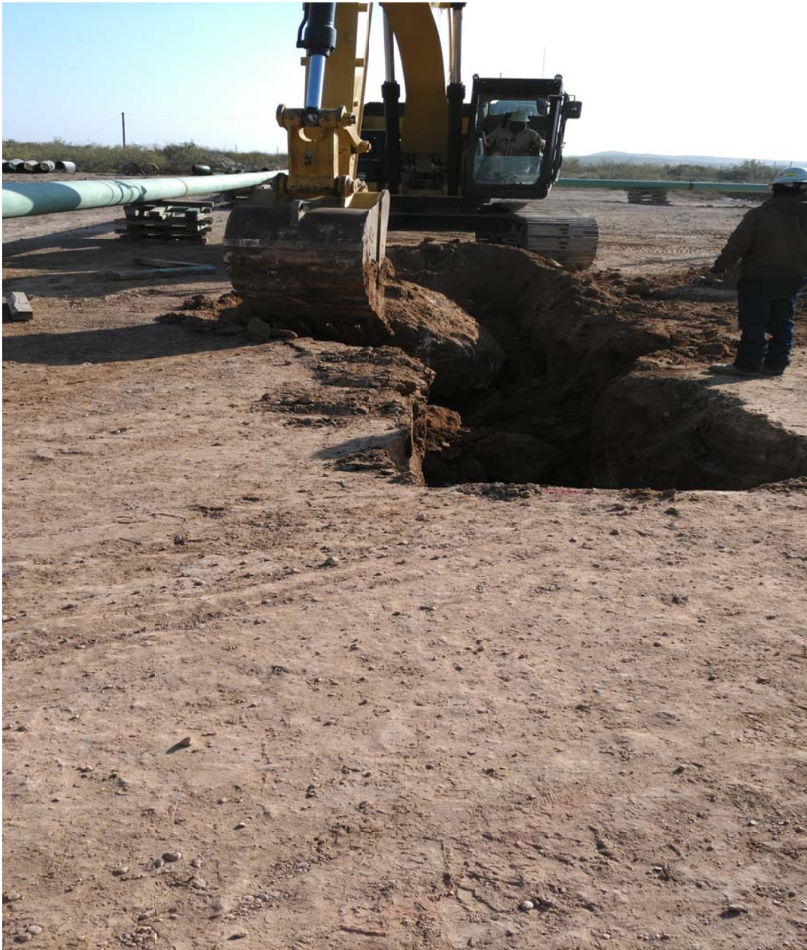
Photo No. 2 – Trenching at Pecos River Compressor Station for the new station piping
