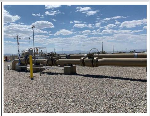
Location: Dragoon Compressor Station Description: Discharge pipelines tie-in yard after gravel and security fencing completed.
