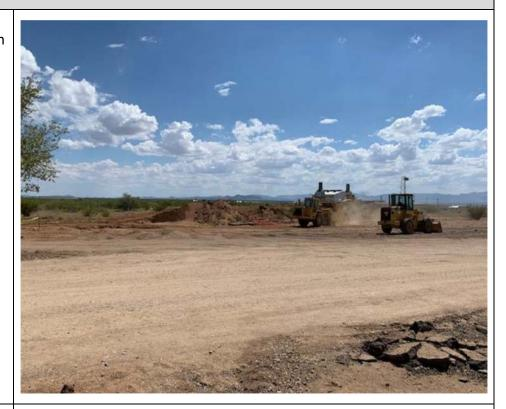
Location: Dragoon Compressor Station Description: Gravel being installed in yard and installation of security fence in background.
