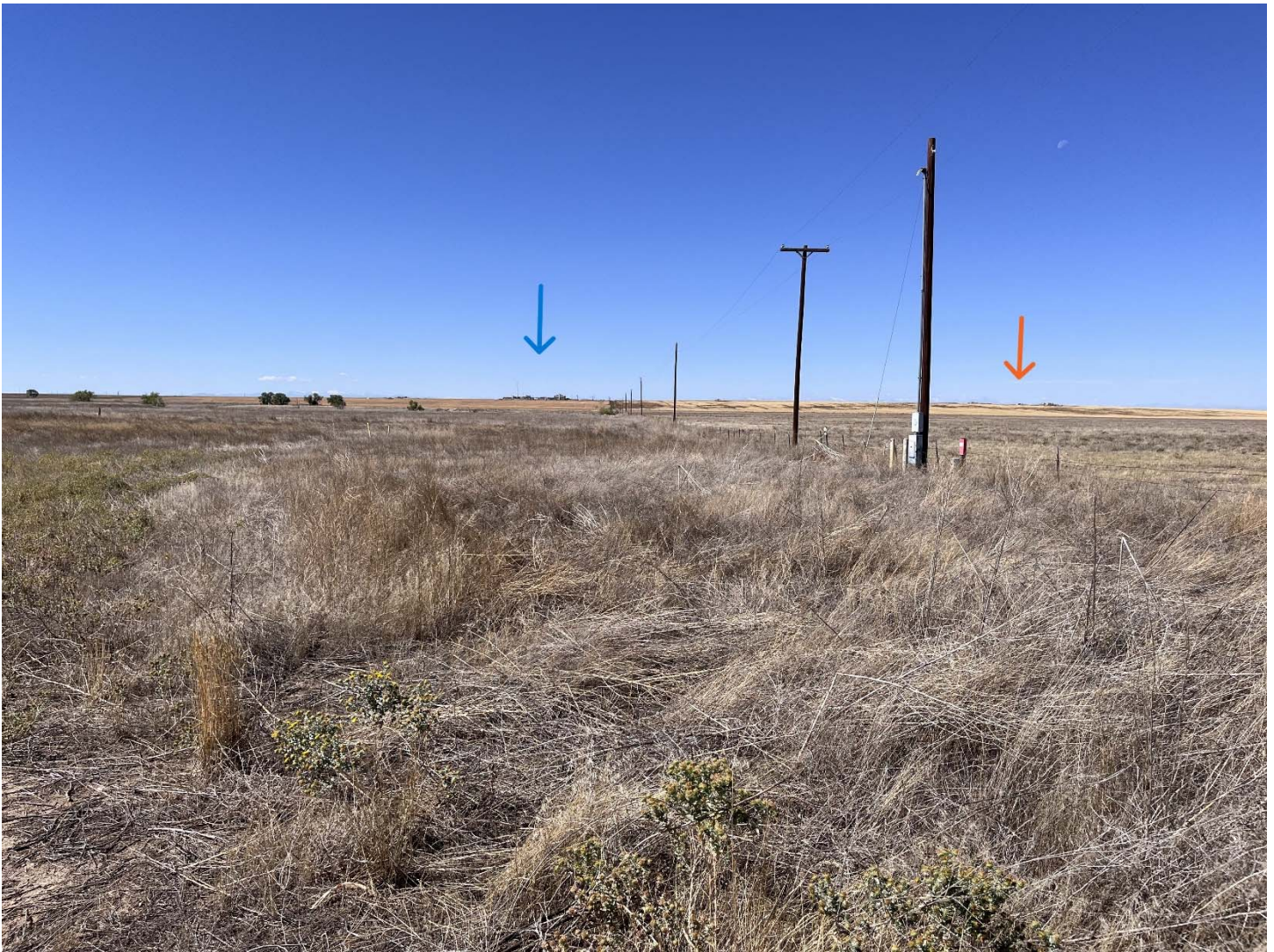
Photo 10-2 – Blue Arrow denotes Compressor Station, Orange Arrow denotes existing injection withdrawal well field north of Compressor Station. Picture taken approximately 1.1 miles east from the Totem Storage Field station facilities.
