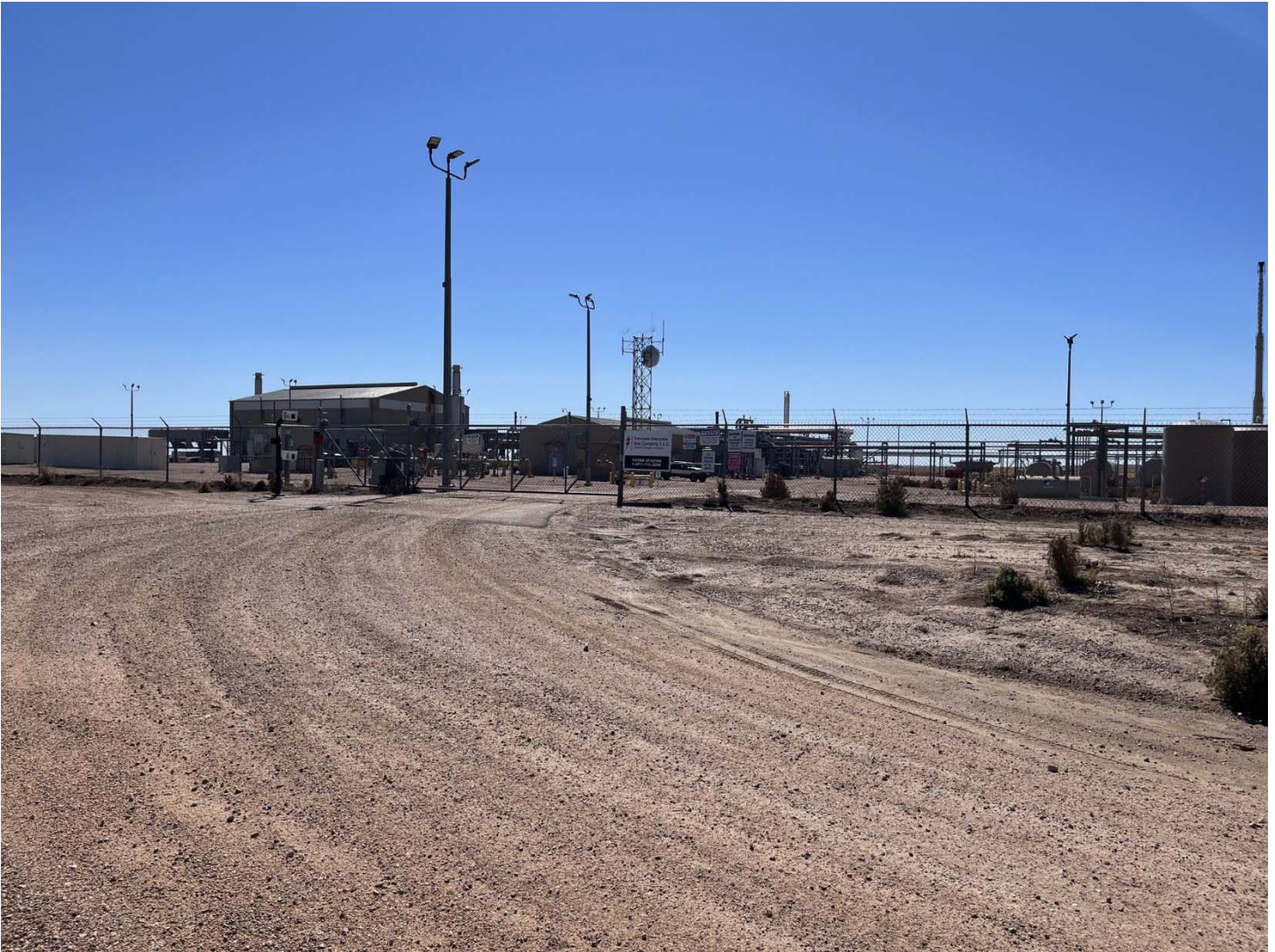
Photo 10-3 – Existing Totem Compressor Station. All proposed modifications will be interior, with no significant modification following construction of the Project.
