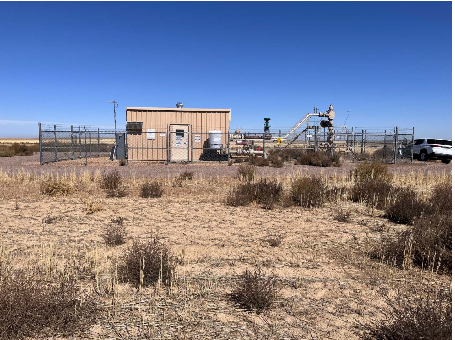
Photo 10-4 - Above Ground Structures associated with Existing Well No. 7. Representative of new above ground facilities to be constructed as part of the Project.
