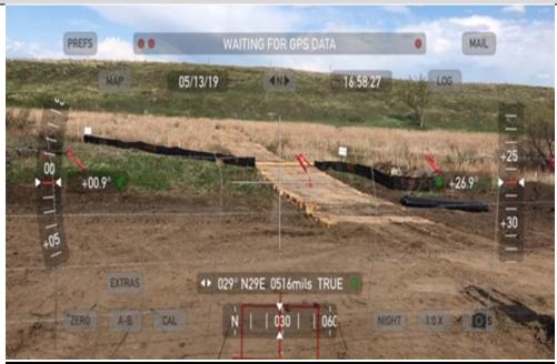
Location: STA 473+92 Direction of Photo: West Description: Silt fence installed at the wetland.
