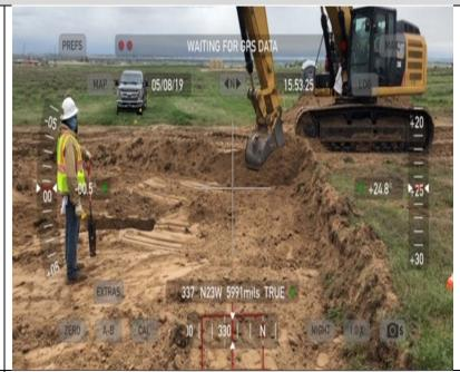
**Location:** High Five Lateral **Direction of Photo:** Northeast **Description:** Contractor placed excavated topsoil on the edge of the extra workspace at MP 0.25
