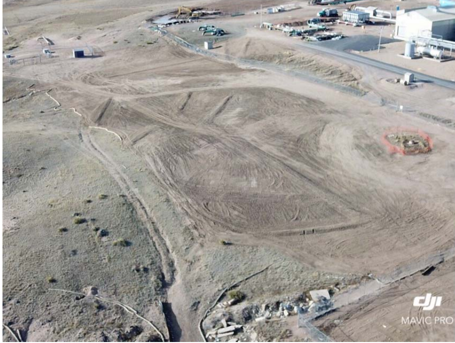
Final clean up
