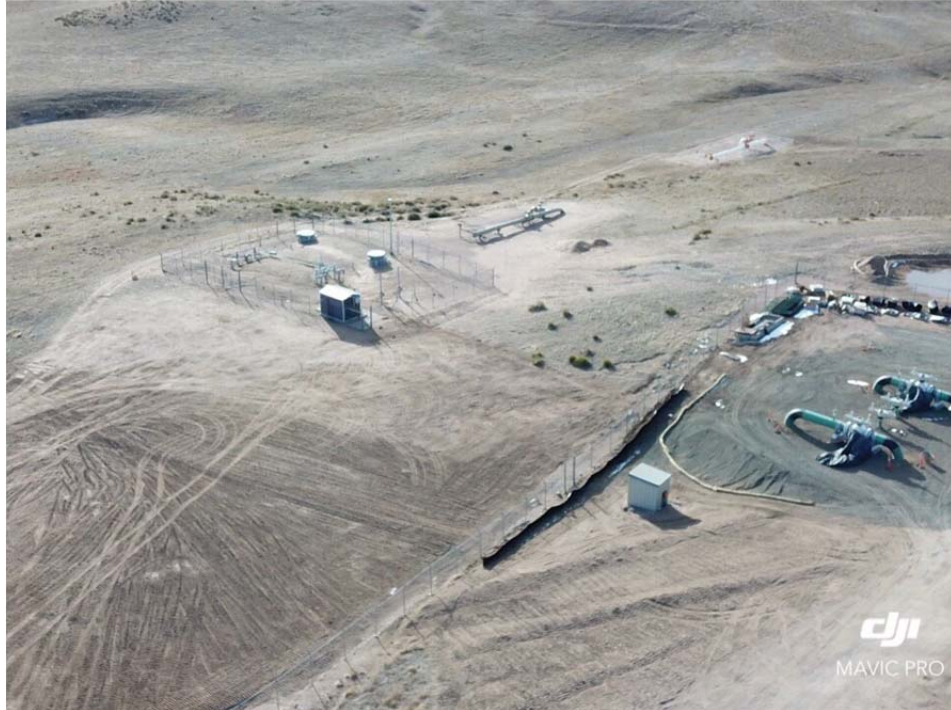
Final clean up
