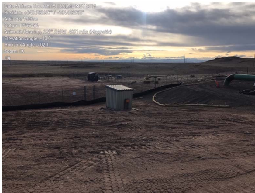
Restored work area east and south of the bi-directional manifold
