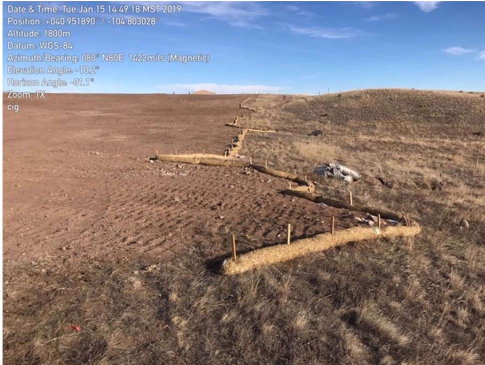
Cleaned up ROW for 24-inch pipeline between CIG and Front Range Compressor Station
