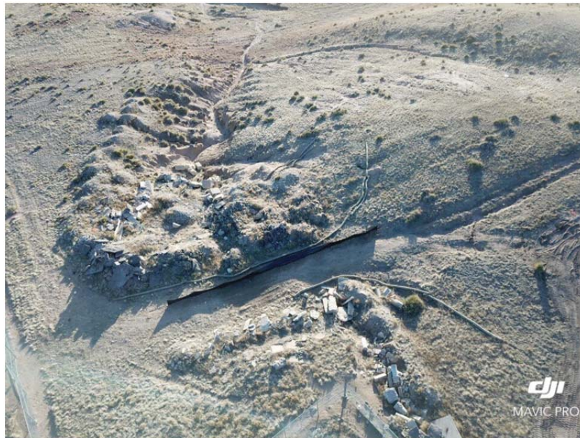
Erosion control installation
