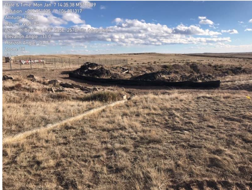
Installed erosion control devices
