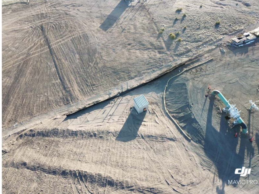
Final grade and erosion control devices
