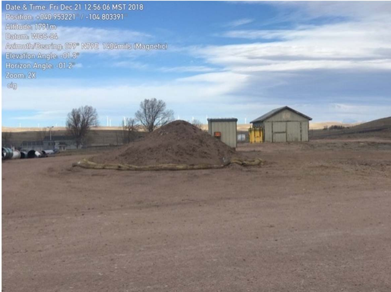
Erosion control around topsoil stockpile
