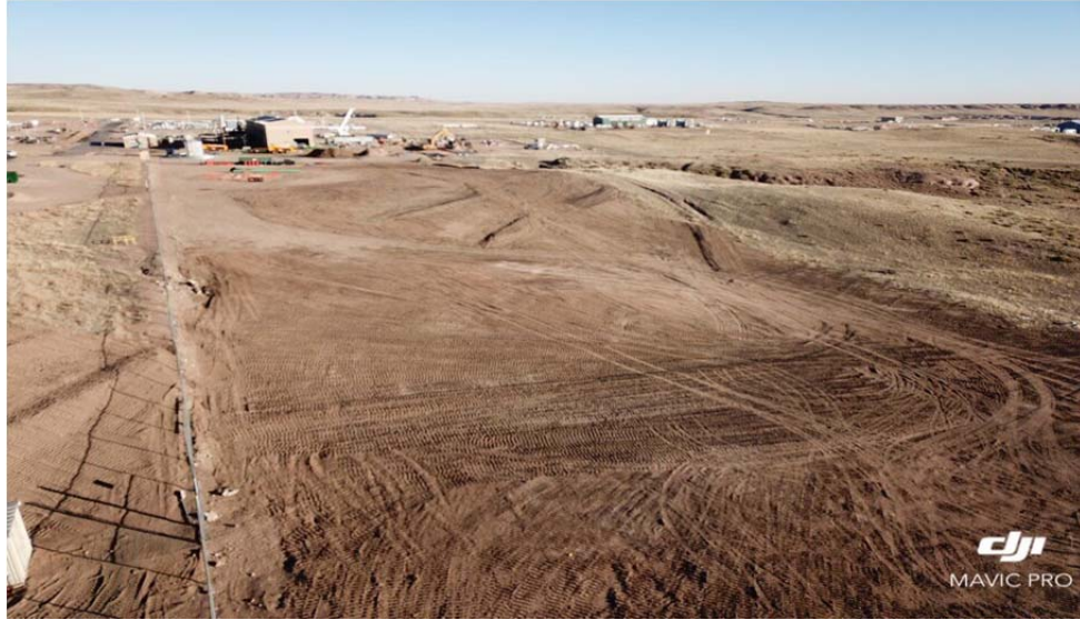
Water bars installed on the 24-inch pipeline ROW
