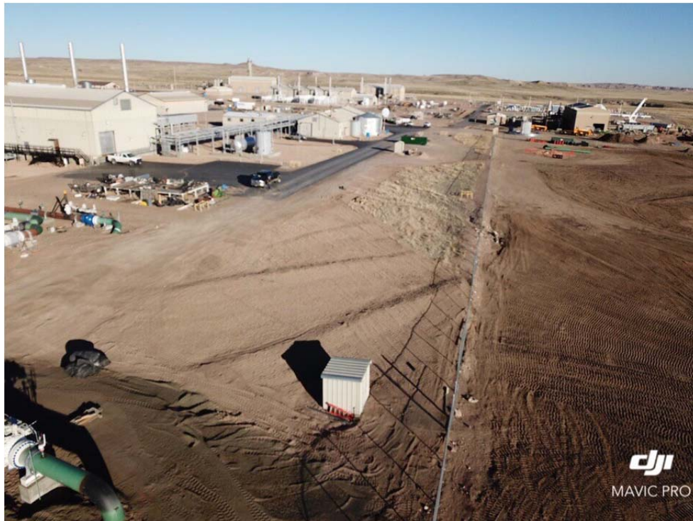
Clean up and water bars on the 24-inch pipeline ROW
