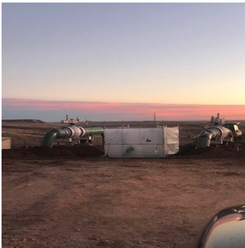
Coating work at bi-directional manifold
