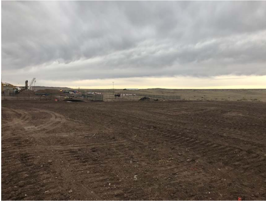
ROW after clean-up
