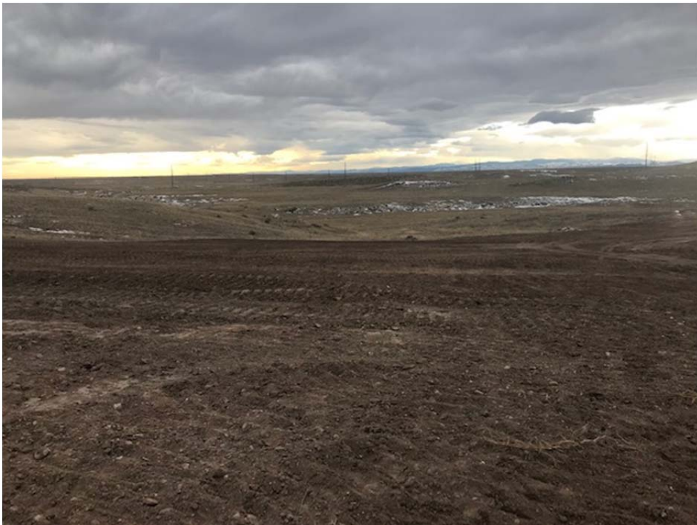
ROW after clean-up
