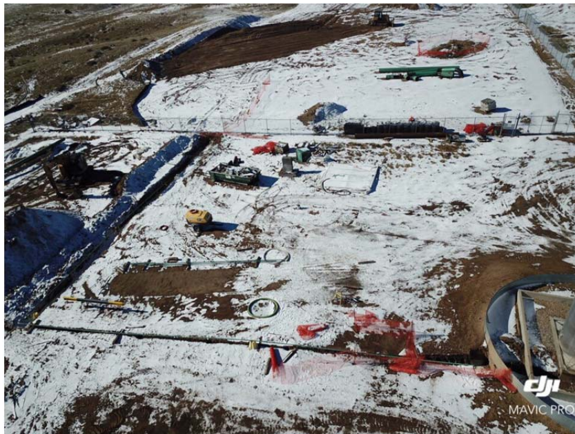
Completed welding of 2-inch drain line
