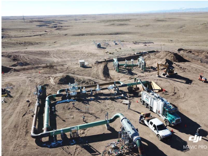
Hydro excavation for installation of pipe supports
