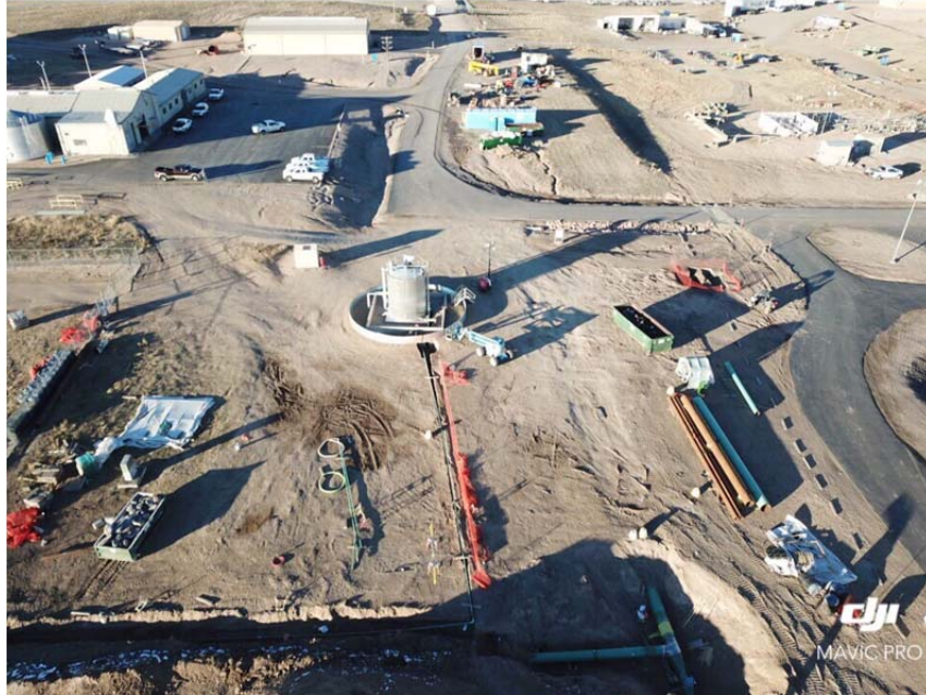
Completed welding of 2-inch drain line
