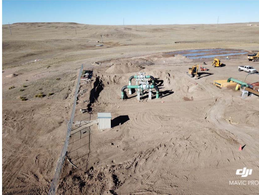
Backfilling the bi-directional manifold
