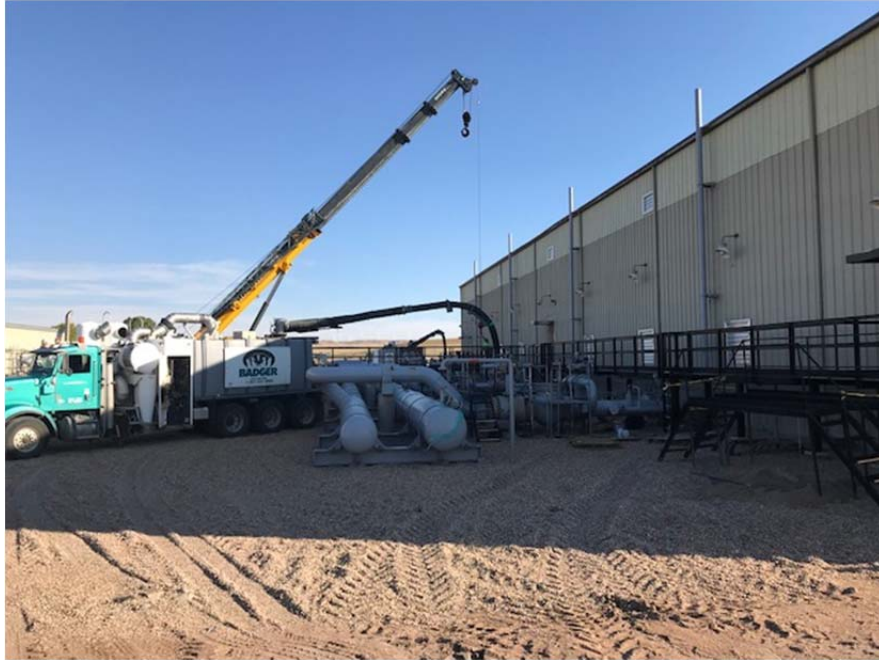
Preparing for hydro test
