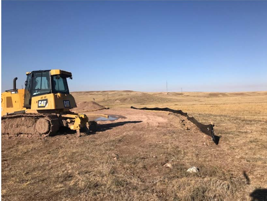
Sediment control devices
